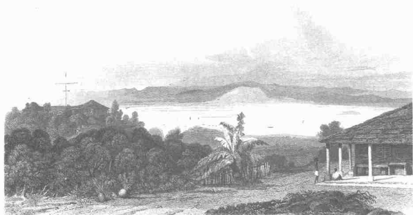
17. Convalescent Bungalow ( right ) and Bel Retiro with its flagstaff ( left ). Note the terraced garden to the right of Bel Retiro, the plinth on which Convalescent Bungalow rested, the building materials, and the servants. (From Captain R. Elliott, Views in India, China, and on the Shores of the Red Sea ... , Vol. 2, 1835.)
