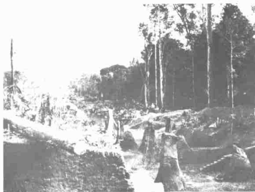
4. Railway construction was greatly hampered by the wet climate and primary rain forest. (From Pat Barr, Taming the Jungle , 1977.)
